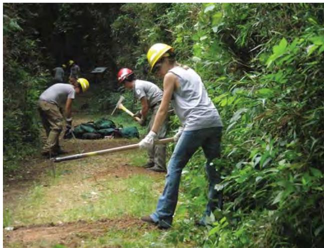
**FIGURE 26.** Trails may require periodic maintenance to fix problems with slough and berm. *Photo courtesy of the National Park Service.*
