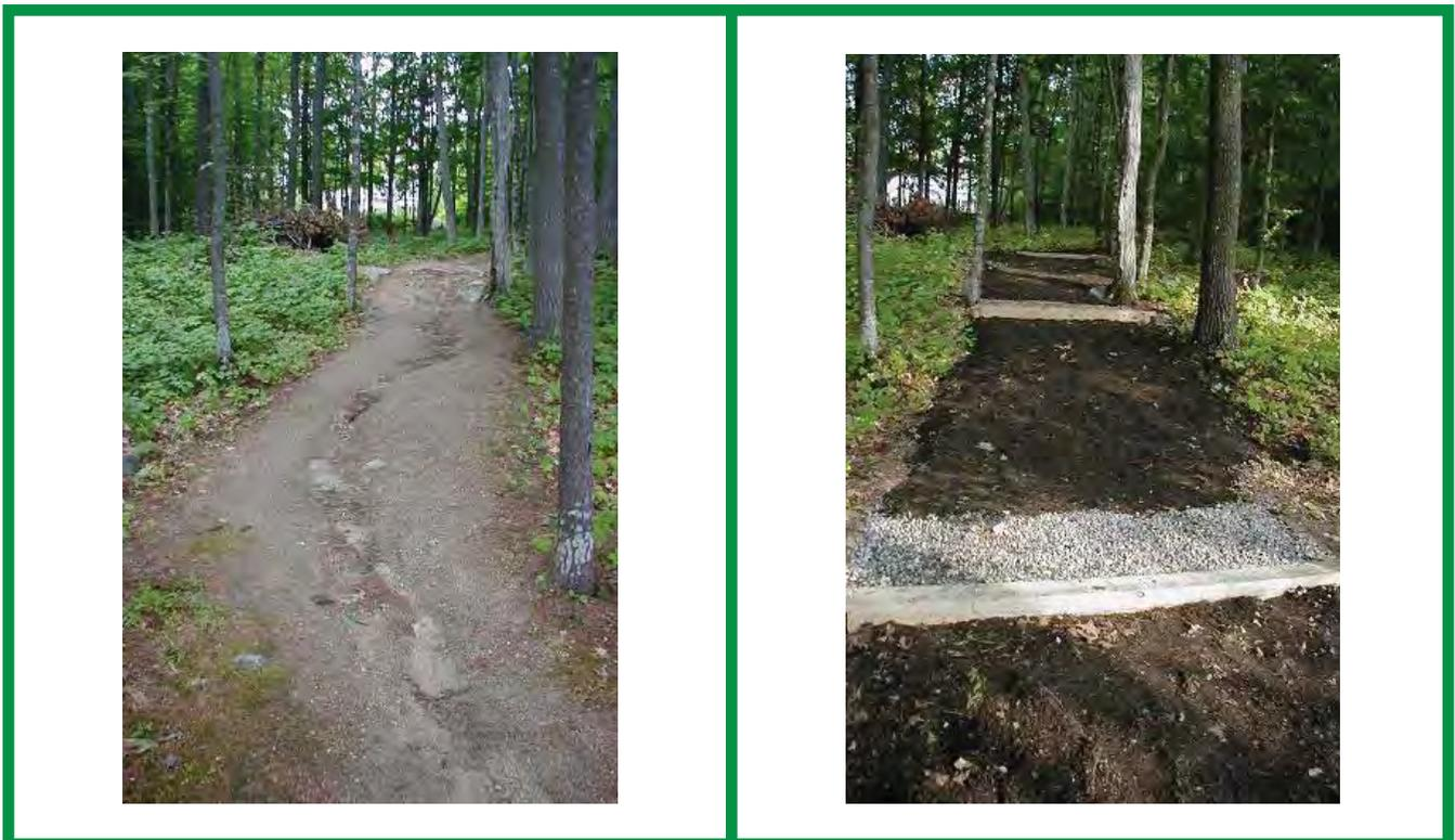
**FIGURE 17.** Trail before and after waterbars were installed to divert water off the tread. Waterbars should be installed only as a last resort. *Photo courtesy of Maine Department of Environmental Protection, Bureau of Land and Water Quality.*
